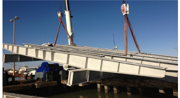
Figure 2 - Fully refurbished section installed
