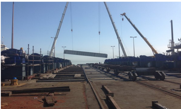
Figure 1 – Removal of platform sections
