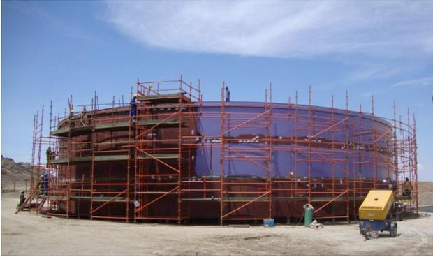
Figure 5 - Second strake in progress
