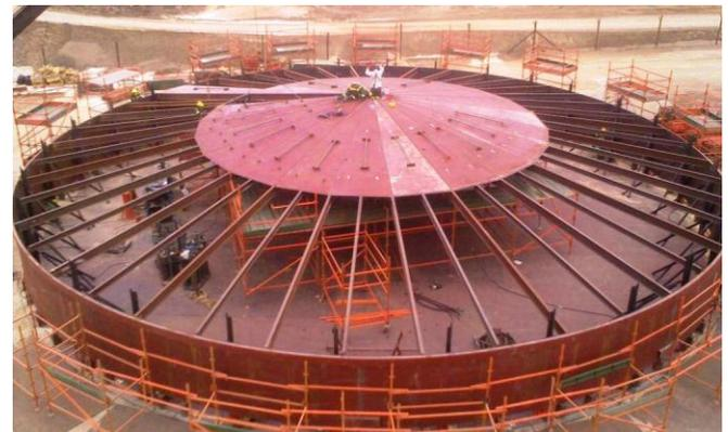
Figure 3 - Roof section assembly in progress
