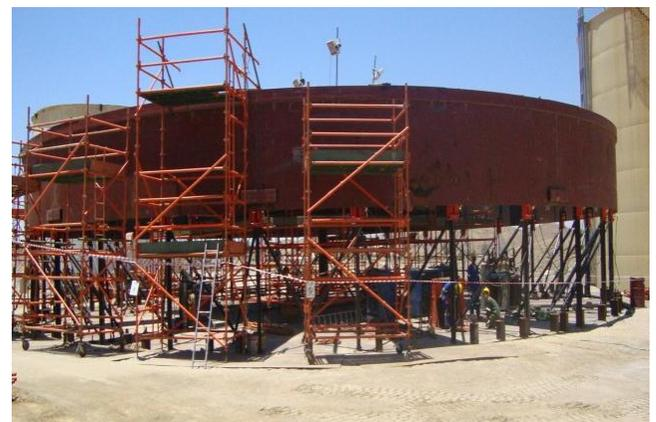
Figure 4 - First strake and roof "jacked up"
