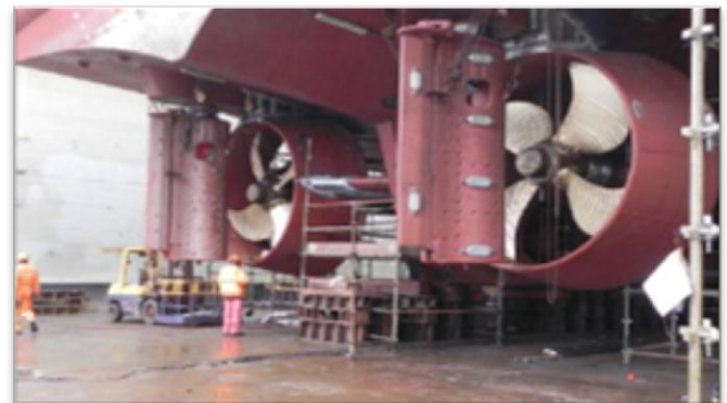
Figure 4 - Kort Nozzles Installed
