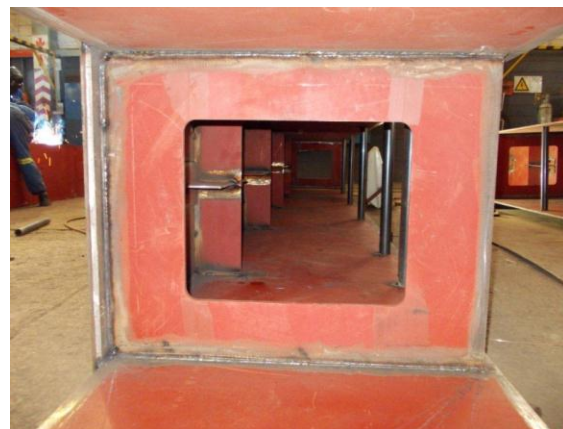
Figure 4 - Internals of bridge walkway during fabrication
