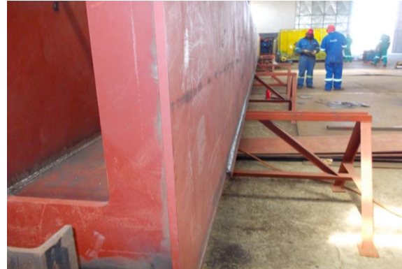
Figure 2 - Bridge walk way
