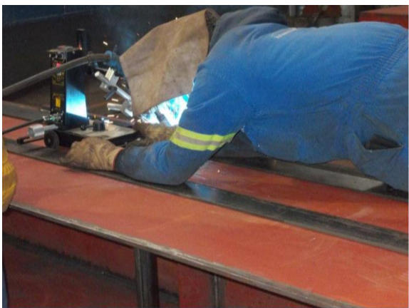
Figure 1 - Welder using semi-automatic welding equipment
