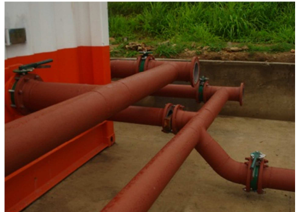
Figure 2 – Assembly and welding of pipes
