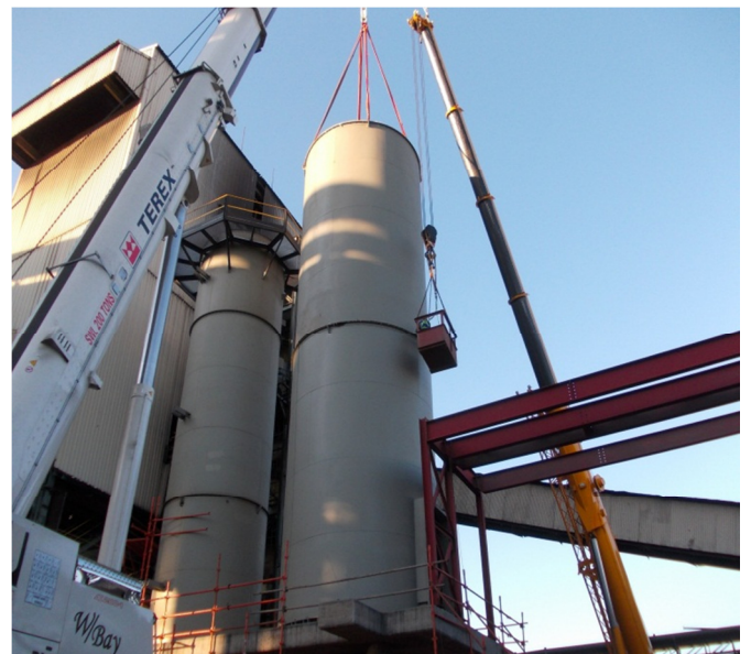
Figure 3 - Tank installed in position
