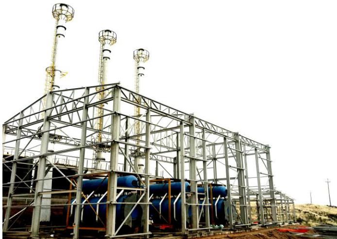
Figure 1 - Starting of project with boilers placed
