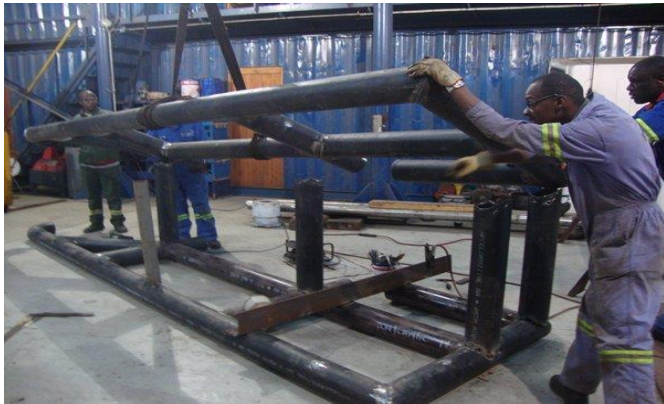
“Assembling in progress”
